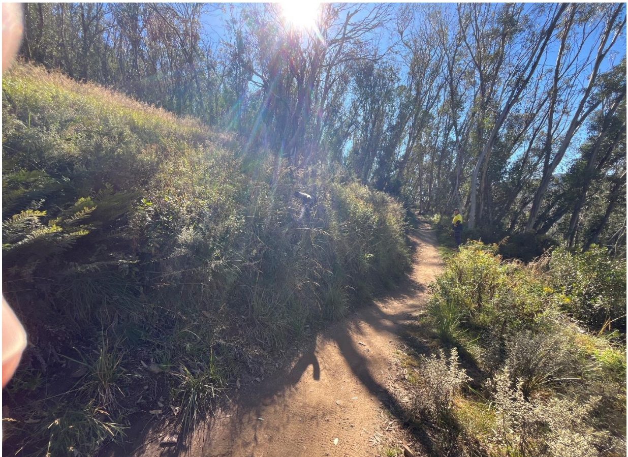
Photo 8: The existing Sidewinder trail be widened on the lower side to avoid encroachment into the Montane Wet Tussock Grassland upslope.
